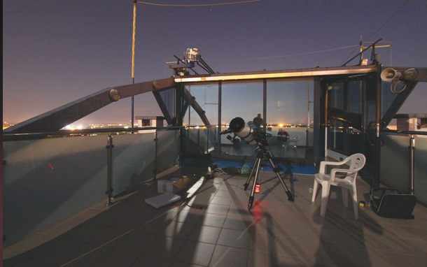
Dome of the Astronomical Observatory of IP UO with a rare sliding roof. Credit: Andrzej Czaiński/IF UO
