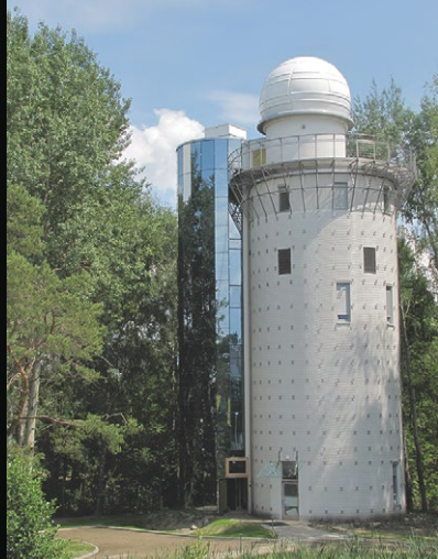
Observatory and Planetarium under construction at University of Bialystok.
