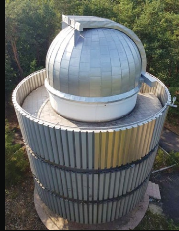
Northern observing station of AO UW in Ostrowik. Credit: AO UW
